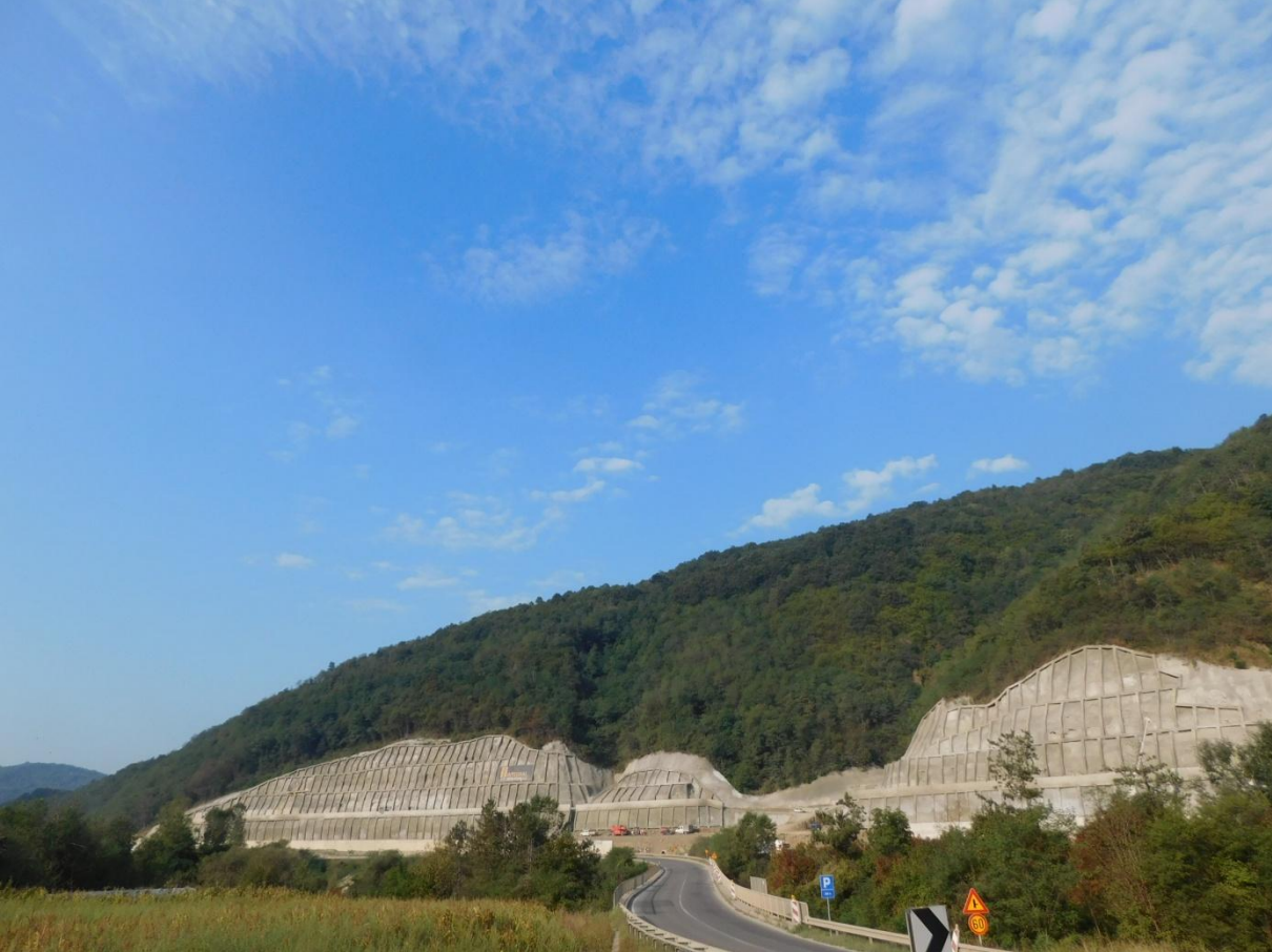
Slope suport project; Grdelica - South Serbia- coridor 10 Diorit supply SDA anchors – Contractor Trace- Bulgaria , subcontractor ; Hyca – Cz 2016/2017
