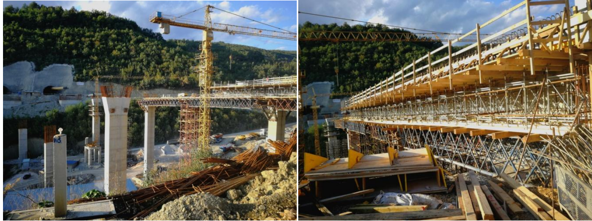
Post tensioning works; OVM system - Viaduct „ Ričice“ –Bosnia and Herzegovina Contractor- Euro-asfalt – Sarajevo – 2017
